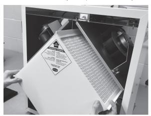
3. Rinse the core with clean water at room temperature (neither cold nor hot).
