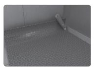
**4** Be sure to leave about 1/4" of space between the membrane and the walls of the room. Measure and cut the membrane to the right length for the room with a retractable utility knife or scissors.
