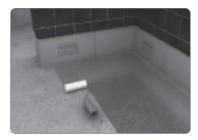
**3** It is strongly advised to use a sealer before installing the membrane.
