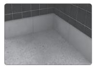
2 Make sure the subfloor is smooth, dry, clean and free of dust. Using a standard SBR-type primer is recommended after cleaning and drying the subfloor.
