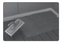
1 Using a notched trowel, spread a layer of flexible tile adhesive over the installed membrane. Take care to avoid pulling the cable out of the membrane. If using tiles smaller than 6" by 6", we recommend to cover the installation with 1/2" of leveling compound first.
