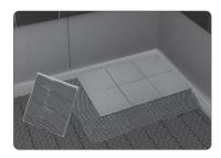
**3** To check the contact with the membrane, lift the first tile to see if it has a good covering of mortar.
