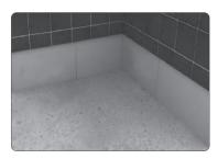
2 Make sure the subfloor is smooth, dry, clean and free of dust. Using a standard SBR-type primer is recommended after cleaning and drying the subfloor.
