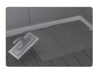
1 Using a notched trowel, spread a layer of C2S-S1-type flexible tile adhesive over the installed membrane. Take care to avoid pulling the cable out of the membrane. If using tiles smaller than 6" by 6", we recommend to cover the installation with 1/2" of leveling compound first.
