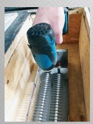
Use the 2 fixing holes in the bottom of the heater to secure it using appropriate screws (not supplied).
